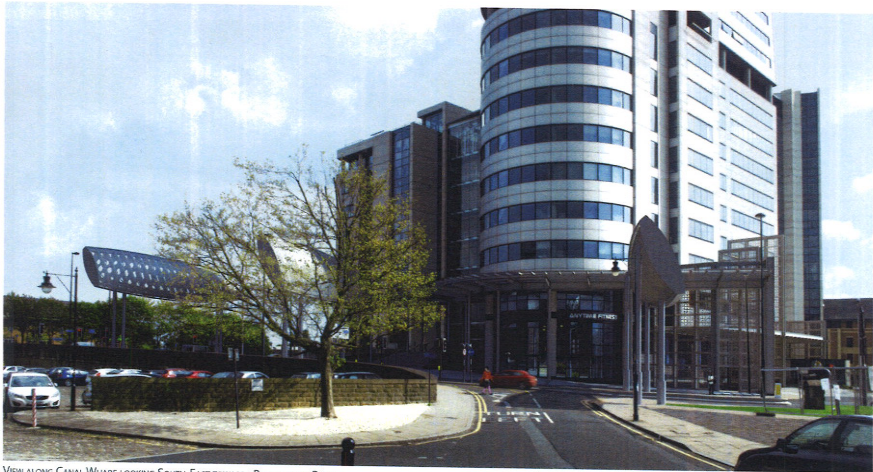
VIEW ALONG CANAL WHARF LOOKING SOUTH-EAST TOWARDS BRIDGEWATER PLACE
